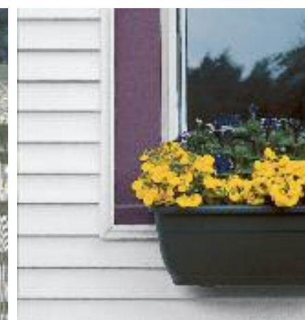
Trimworks custom crown molding used with wood window trim.
