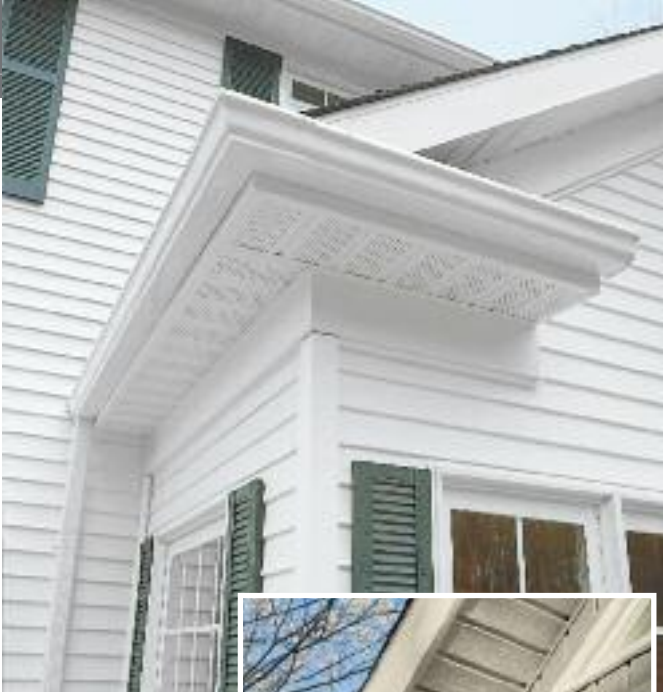
Beautifully vented panels provide continuous airflow to help cool attics (above).
