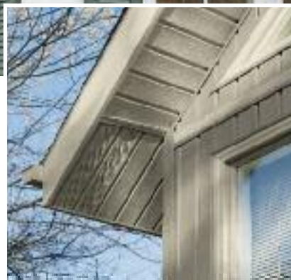
Beautifully vented panels provide continuous airflow to help cool attics (above).
