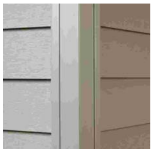
Traditional corner post with foam insert.
